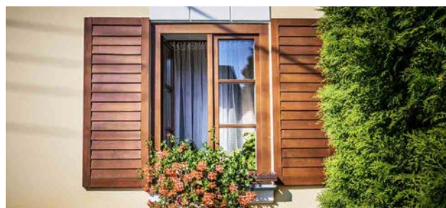
WINDOWS AND DOORS
