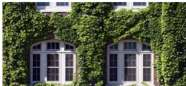
WINDOWS AND DOORS
